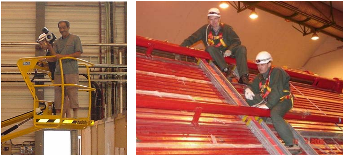
Fig. 10. Geometrical survey (left) and cabling activity (right) at ALICE
